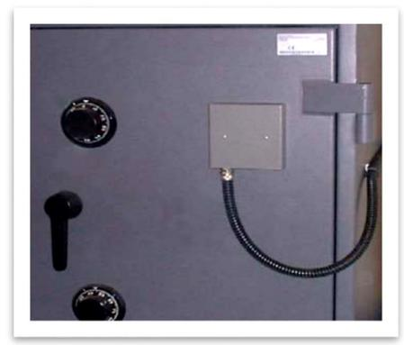
The LFS (Low Frequency Stress) Attack detector series, outputs an alert after analysis of the pressure and noise generated within the structure of the protected area, virtually ignoring localised noise and general vibration. The combination of the following conditions are detected by the analyser.
